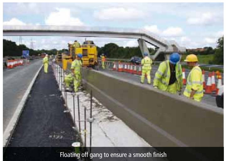
New Britpave Step Barrier & Drainage Channel
